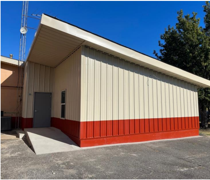
Pictured Above: The continued remodeling of station 4.
